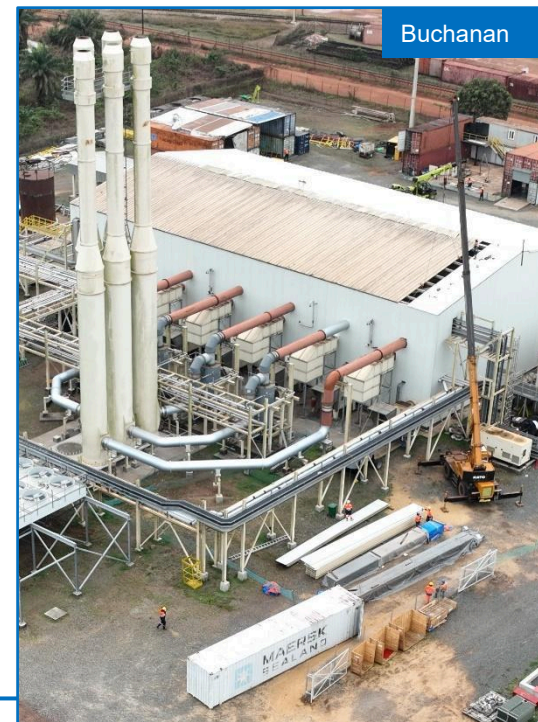
~100 MW power being generated with 10 engines at Tokadeh and 5 engines at Buchanan
