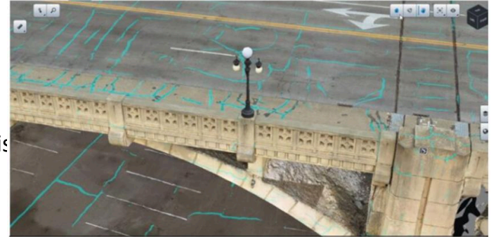
Robert Street Bridge shown highlighted with digital road markings after an inspection. Image courtesy of Collins Engineering.
