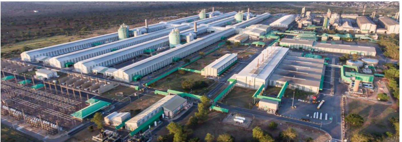
Figure 5.6b Industrial park infrastructure supporting manufacturing, logistics, and export-oriented investment in Mozambique. Photo: MozParks.
