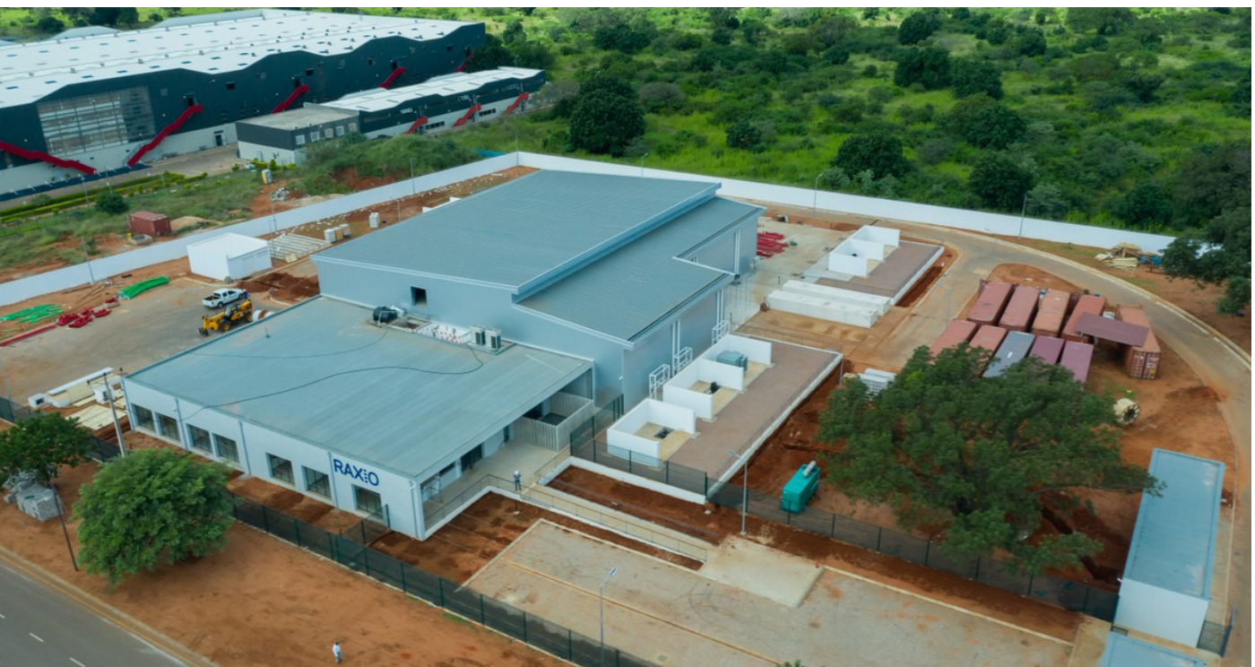
Figure 4.5 - Mozambique’s first Tier III carrier-neutral data centre, located in Beluluane Industrial Park, is helping position the country as a regional digital infrastructure hub. Photo courtesy of Raxio Data Centres Mozambique.
