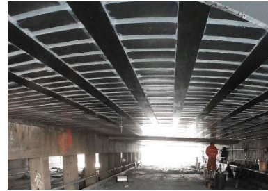
Steel plate reinforcement
