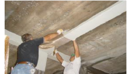
Textile reinforced mortar
