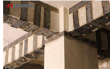
Steel plate reinforcement
