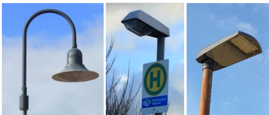
Fig. 6: Left: these “bell-shaped” luminaires are full cut-off and the lamps had been replaced to 2200 K lamps. Middle: these “Koffer” luminaires were replaced by fully shielded 2200 K luminaires (photos: A. Hänel)
