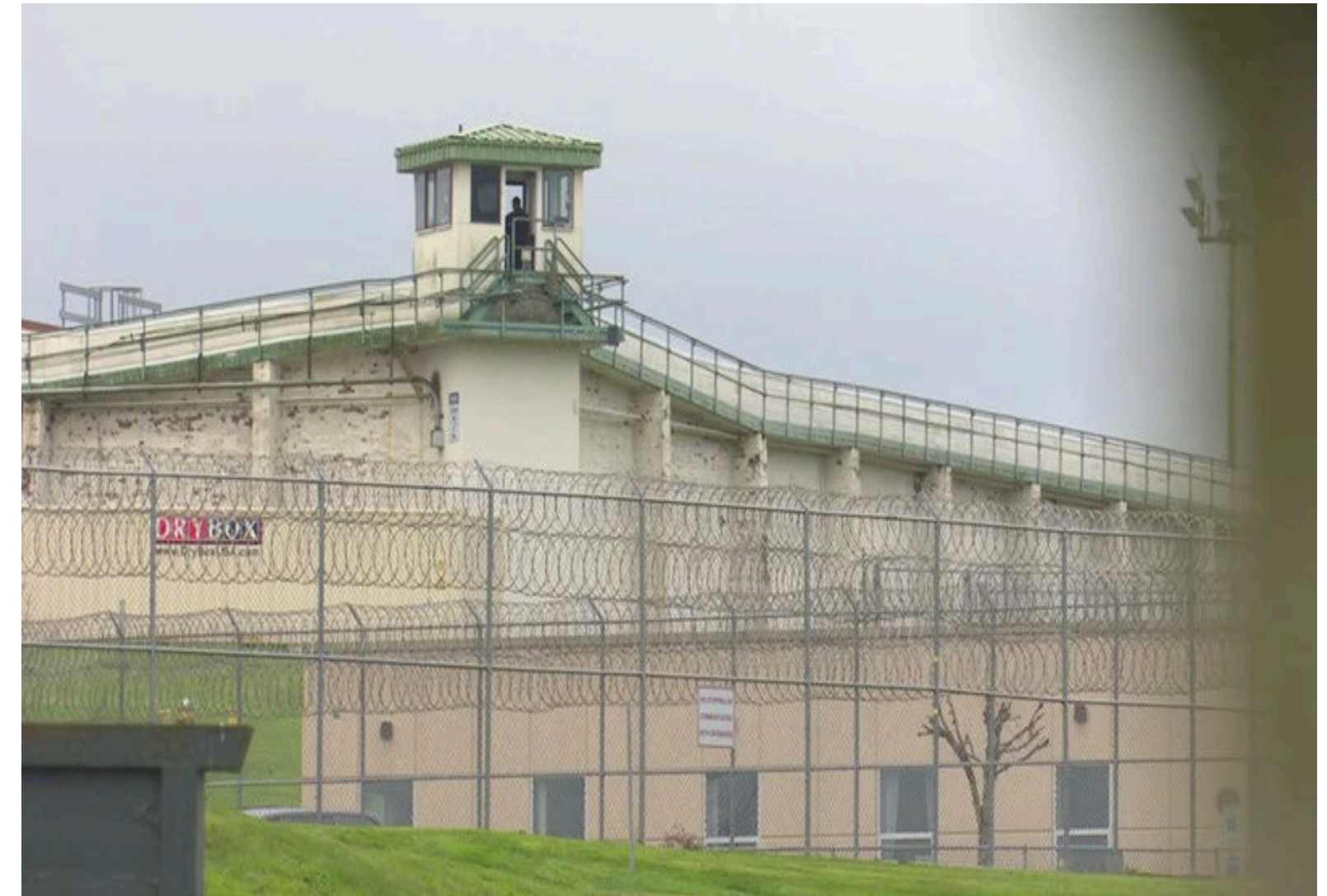
Large DBB project at MCC to remove and replace 120-year-old perimeter wall.
