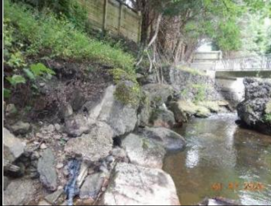
Evidence of bank erosion near properties/under-scour at Gabions
