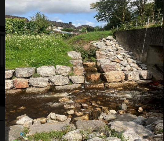
Tumbling mountain stream cascade to create interest, control velocities
