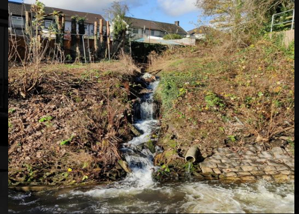
Undefined stream entry creating local erosion
