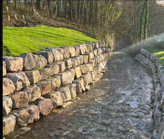
Sustainable blockstone bank stepped back to create habitat potential, designed to stabilise A4119 and extreme storm events
