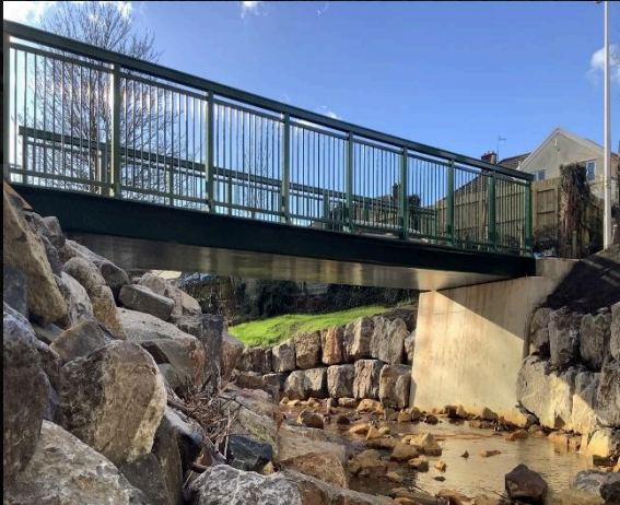
New Active Travel Bridge (11.5m span by 3.5m wide) designed with innovation in mind
